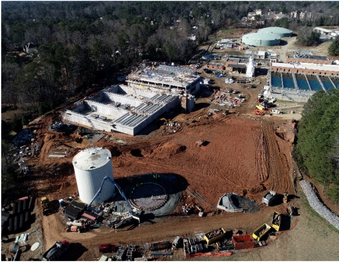
Aerial view of construction progress as of December 2019
