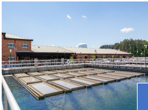
Wyckoff Water Treatment Plant
