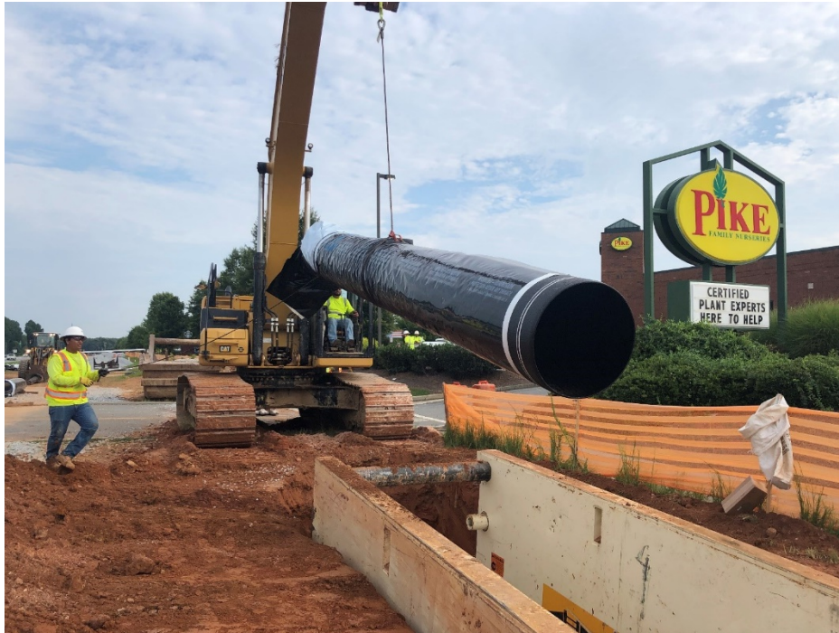
Pipeline being laid along U.S. Highway 41 in Acworth
