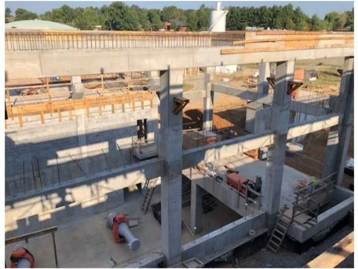
Construction of Filter Building
