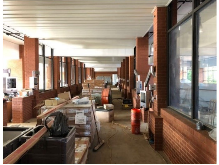
New Quarles Plant 1 filter gallery, under construction
