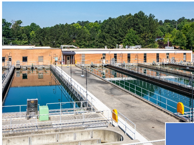
Quarles Water Treatment Plant 2
