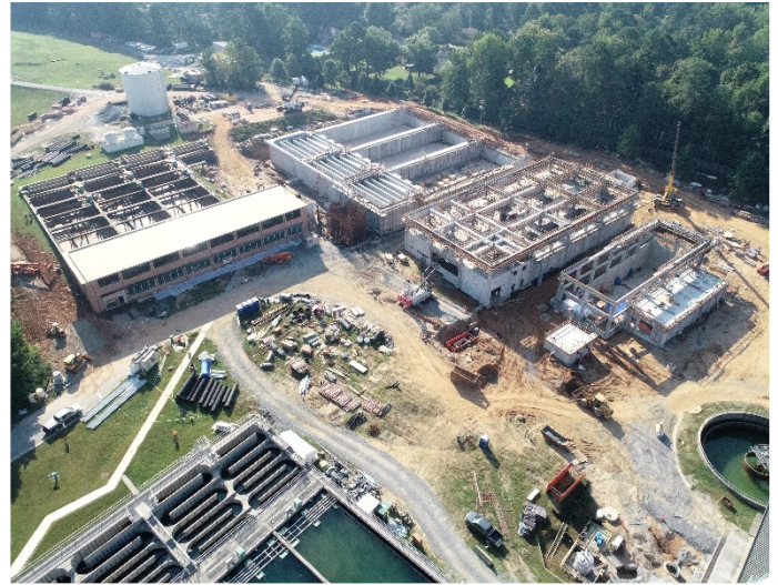
Aerial view of construction progress before the old Quarles Plant 1 (on left) was completely demolished
