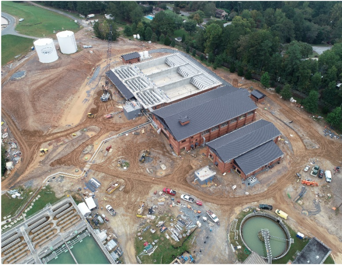
Aerial view of construction progress as of November 2020
