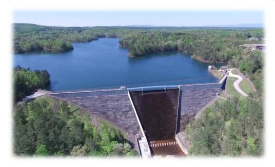
approximately 411 acres and impounds 5.7 billion gallons of water. The reservoir is jointly owned and operated by CCMWA and the City of Canton, with CCMWA owning 75% of the project. The reservoir was constructed with a designed yield of 44 million gallons per day (MGD), with 33 MGD allocated to CCMWA.
