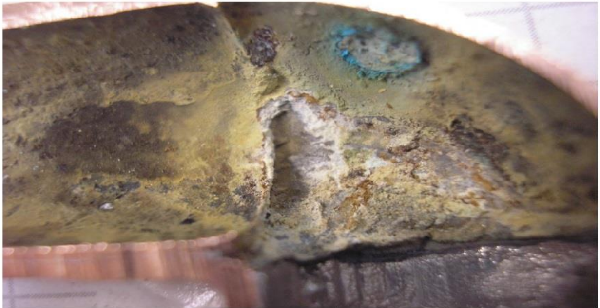
Figure C6: Resident G joint sample. Note: this is a good example of corrosion damage done by excessive solder and flux application.
