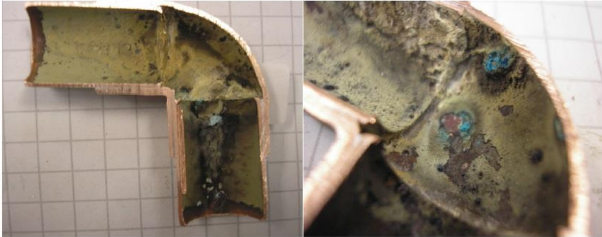
Figure 5: (G Specimens) Pipe joints showing incomplete solder penetration (wicking) into the crevice between the tubing and the connector, un-reamed tubing cuts and excessive flux and solder application. Note: carbon residue from the original flux application is still present on these surfaces.
