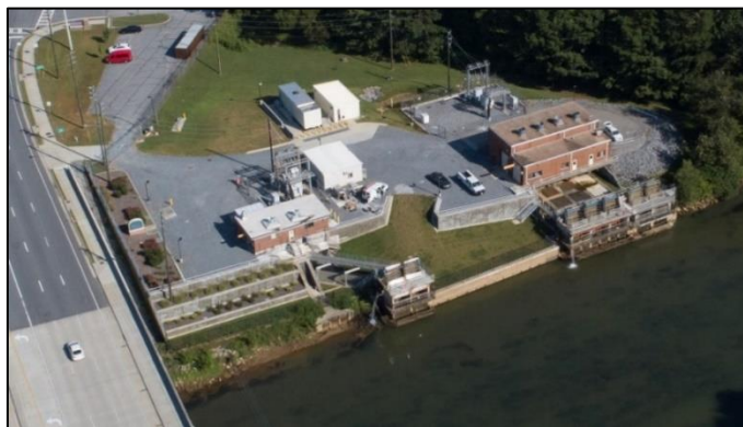
Quarles Water Supply Pump Station
